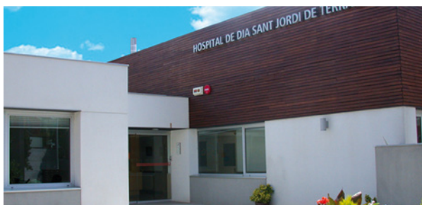
Hospital de Dia Sant Jordi
