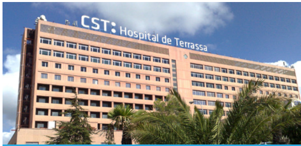
Hospital de Terrassa
