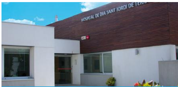
Hospital de Dia Sant Jordi
