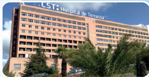
Hospital de Terrassa
