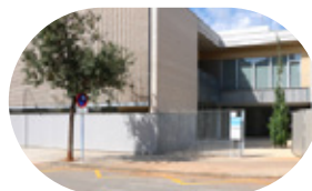
CAP Can Roca Terrassa
